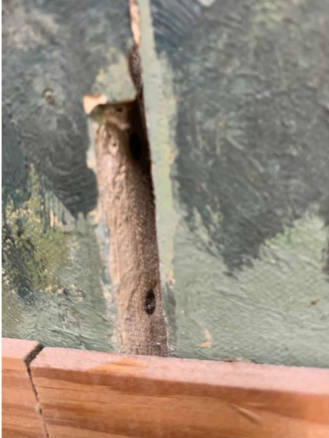
Detail of gap created by bowing strainers and uneven seam
