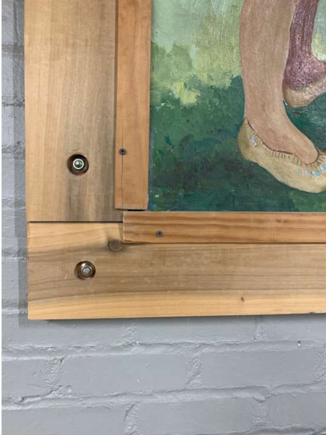
Detail of 2"x6" wood collar and strips used to mount mural to wall
